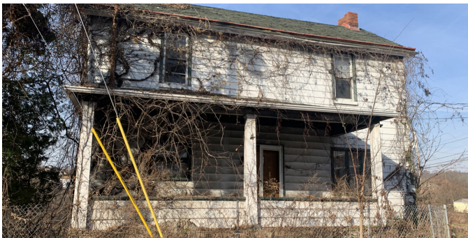
Blighted Property in Monessen Source: Westmoreland County Planning
