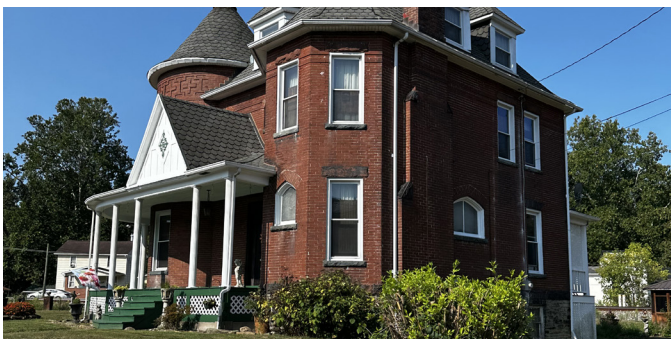
House in West Newton Source: Westmoreland County Planning
