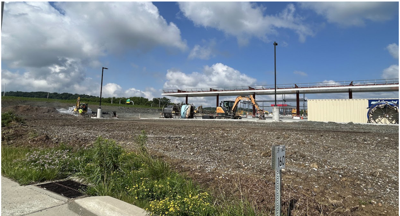
Rutter's Construction at Commerce Crossing Source: Westmoreland County Planning
