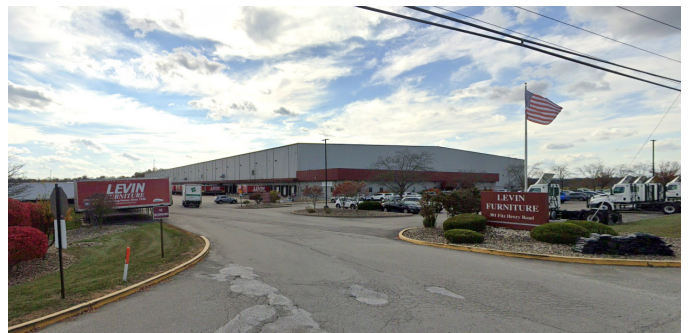
Levin Warehouse, South Huntingdon
