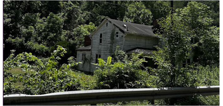
Blighted Property in Smithton
